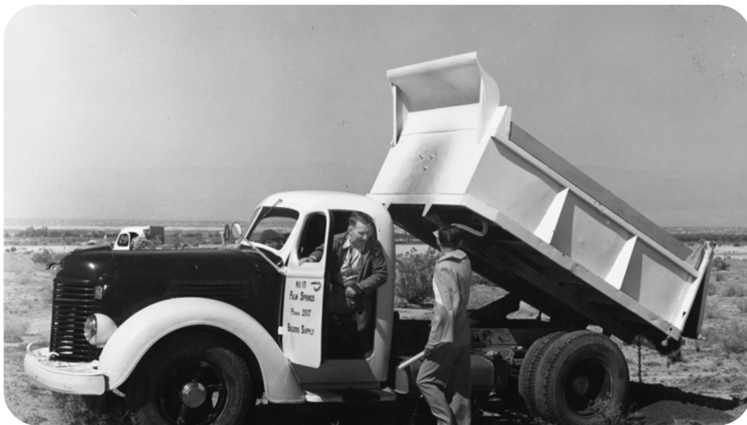
Truck dumping the first commercial dirt in July 1946.
