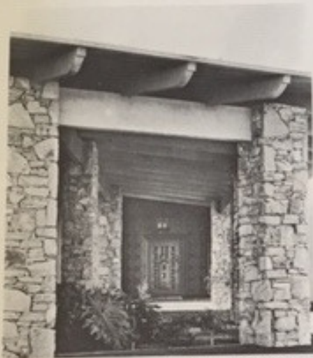
The beautiful La Muir Terrace home of Mr. and Mrs. Louis Tashman served President Lyndon B. Johnson as his Desert White House recently. The 10,000 sq. ft. house has a total roof area of 18,000 sq. ft. Wide expanses of glass allow the Tashmans' uninterrupted views of a wide segment of the desert. Other features of the house are the generous use of carefully selected Ponce Verde stone laid without mortar, 16' ceilings and the beautiful hand carved front door.
