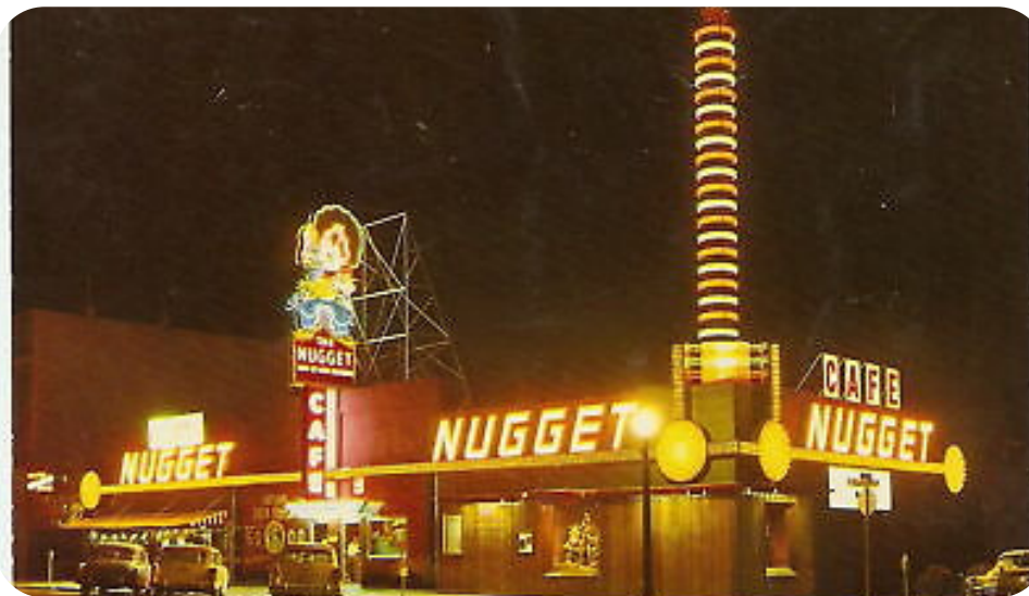
The Nugget Casino (1950s), Carson City, NV
