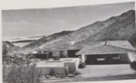
The Thomas Grilling hilltop residence in Southridge designed and built by Patten-Wild, Inc. Perlette marble was used throughout the large entry hall and dining area in this fine home. Views of the golf courses below and wide swms of the desert as far as the lower end of the valley can be seen from the large curved window at the dining room.
