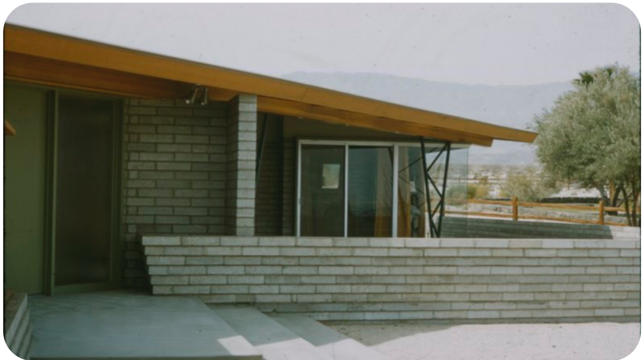
Construction photos 1953/4: UCSB Archives
