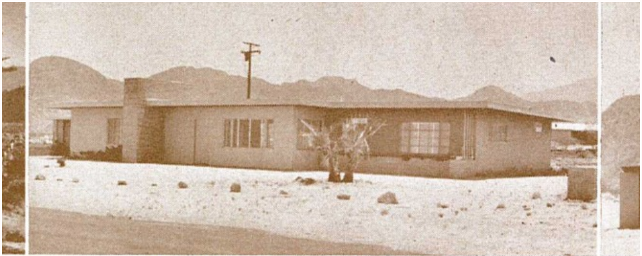
Mr. and Mrs. Charles McVey's new home is typical of much of the smart new building.
